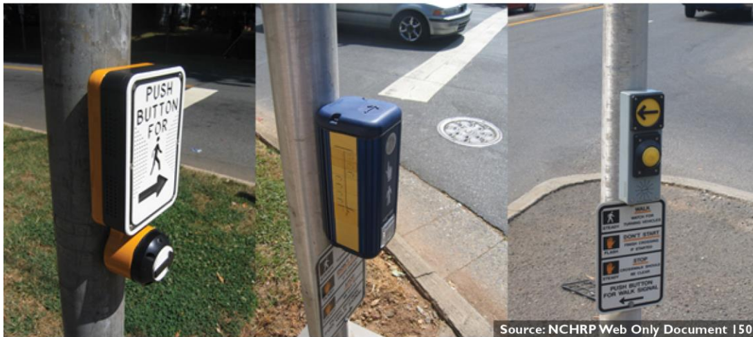
Accessible pedestrian signals
