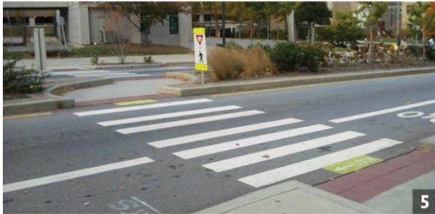
Marked crosswalk with refuge and supplemental devices
