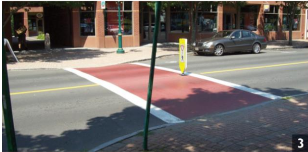
Marked crosswalk with supplemental devices
