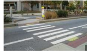
Marked crosswalk with refuge and supplemental devices
