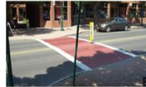
Marked crosswalk with supplemental devices
